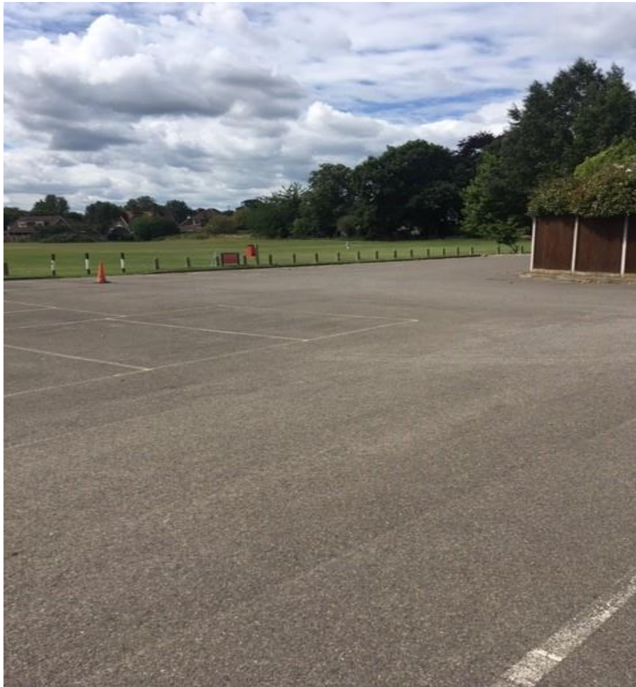
Slide 10 – car park looking west
